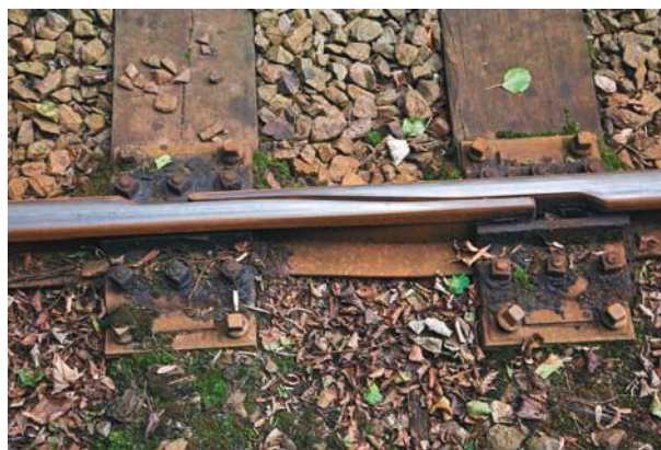
Figure 19.2a Tapered overlap of rails
