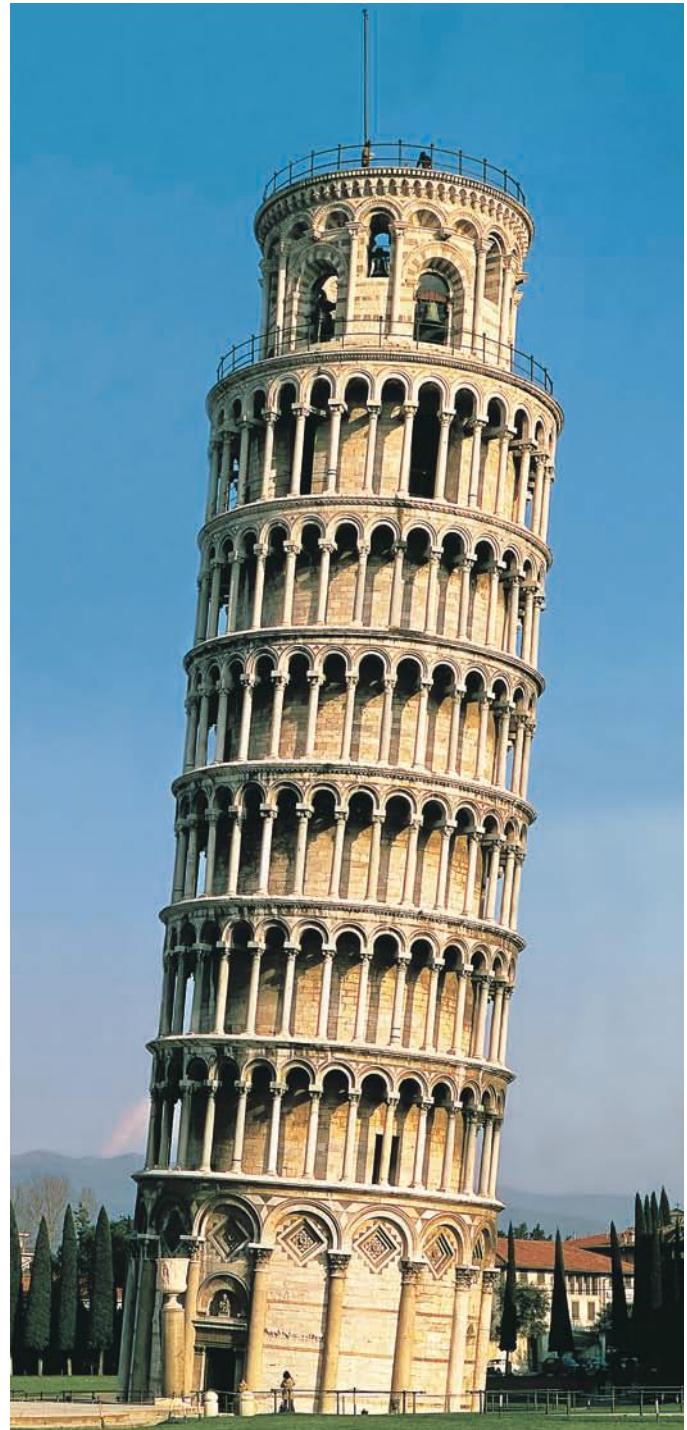
Figure 4.2 The Leaning Tower of Pisa, where Galileo is said to have experimented with falling objects
