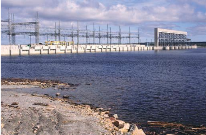
Figure 15.3 Tidal barrage in Canada
